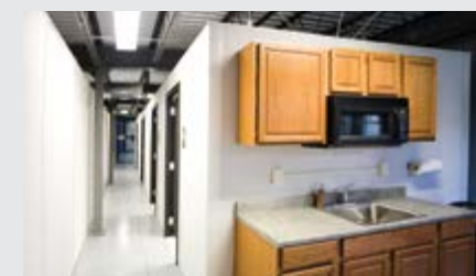
Vinyl Faced Wall Panels partitioning administrative offices
