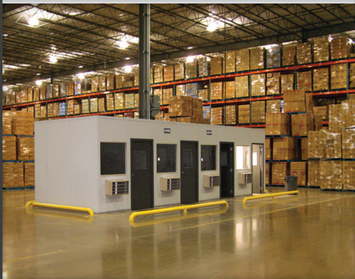
Four, warehouse management offices; constructed of InPlant's Standard Steel System & 3\"
