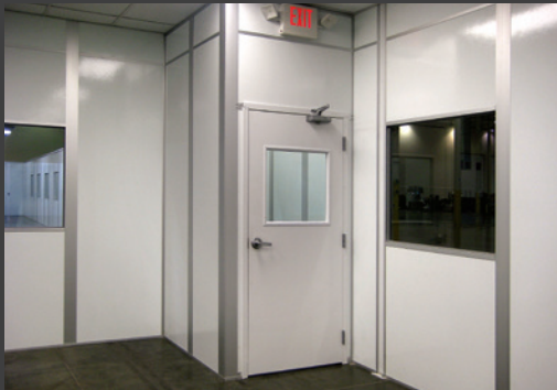
Temperature & contaminant controlling entrance, 3" Aluminum System & FRP Faced Wall Panels
