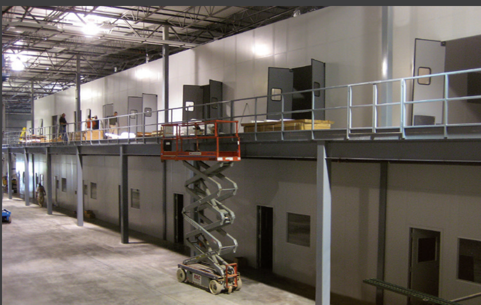
Warehouse storage over lower production rooms, 3" 16 gauge Heavy-Duty Steel System & tall Wall Panels
